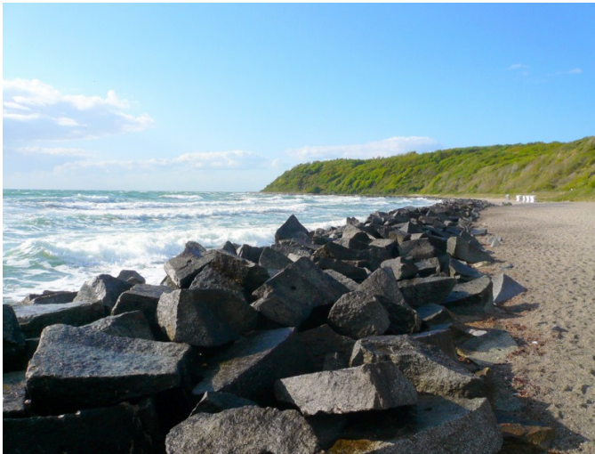
7. Protecting stone blocks
